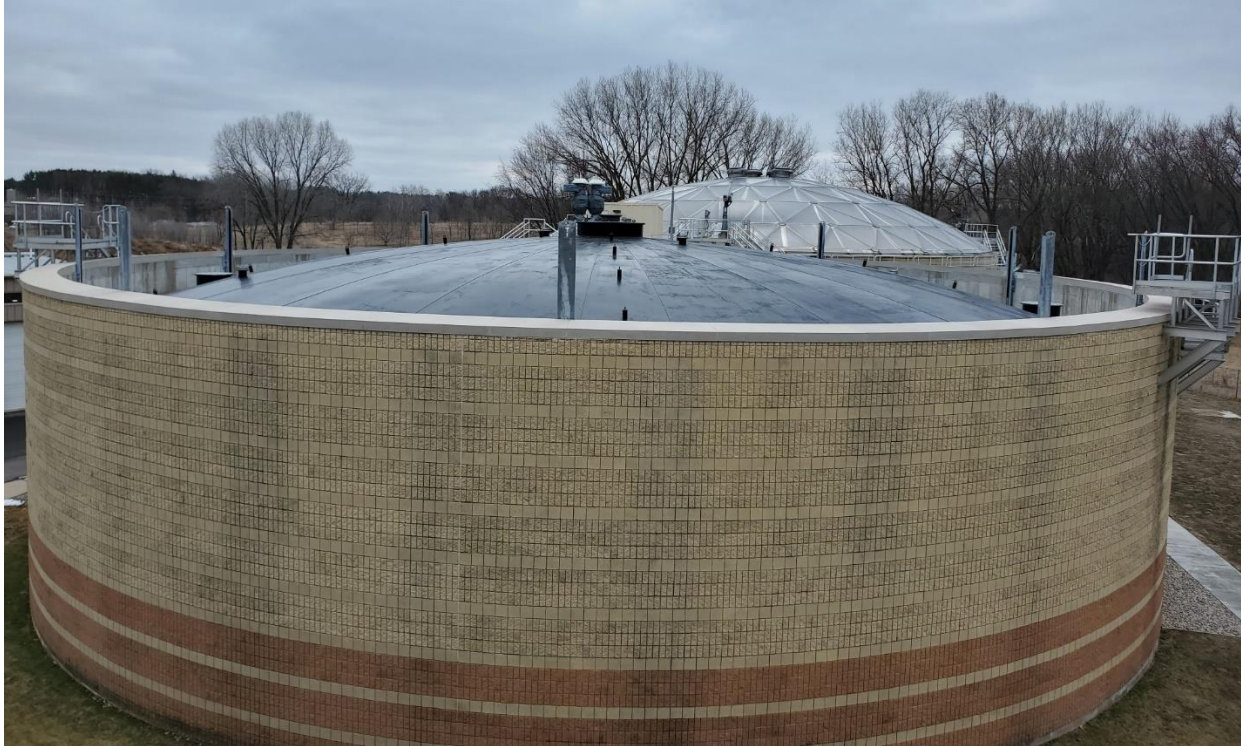
Figure 3. New 1.5-million-gallon anaerobic digester, converted from a wastewater solids storage tank in 2018. Source: City of Stevens Point.
