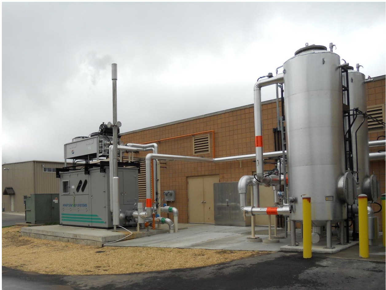
Figure 1. 180-KW Cogeneration engine and hydrogen sulfide removal tanks. Source: City of Stevens Point.
